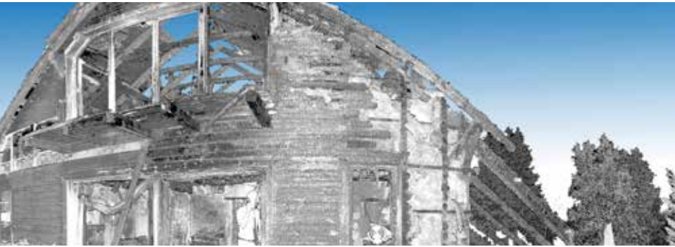
3D point cloud of a burnt restaurant
