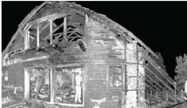
3D point cloud of a burnt restaurant
